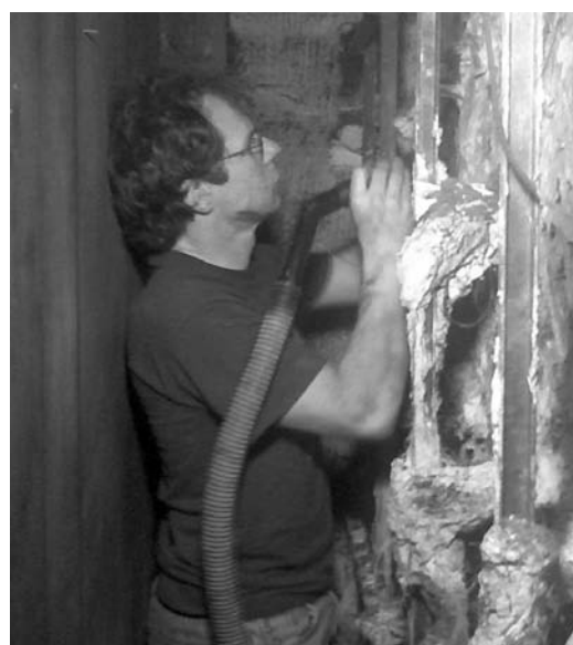
While the swell shades are removed for bearing lubrication, Larry Mayer takes the opportunity to remove extra plaster from the inside of the decorative grilles to hopefully improve tonal egress
