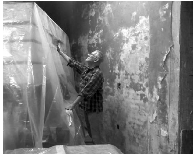
Bob Zat finishes plastic-wrapping pipe crates and chests so that plaster repair work can begin
