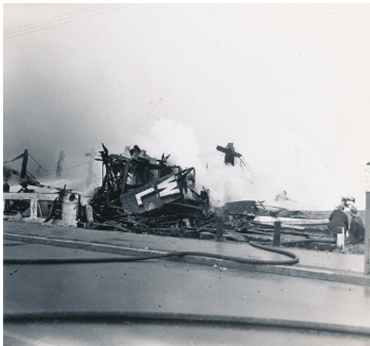
Near total destruction, only W and L remained of the landmark ROLLERBOWL sign
