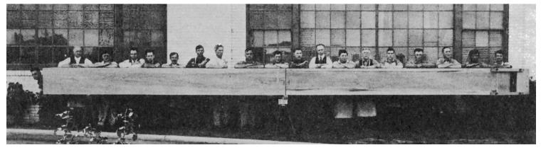
Thirty-two foot Open Diapason pipe, on display in the Morton factory driveway, was the largest pipe constructed for the 85-rank Morton installed in the University of Southern California Bovard Auditorium in 1921. Pipe was 31' 3" long. Note man peering from left end of pipe.
